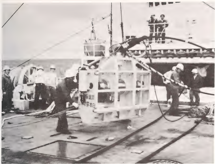
Figure 10 Trial Layings of the Terminal Apparatus
